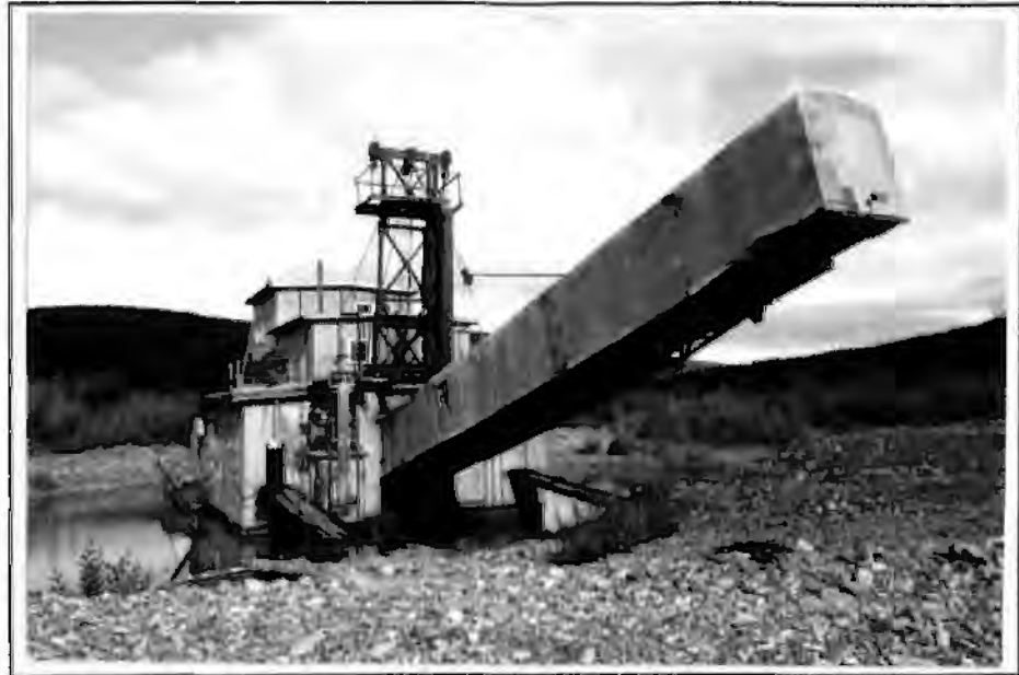
Figure 70. The Matheson Dredge, 1993. The view is looking northwest.
